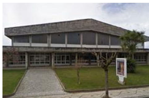
Figura 70 – Pavilhão Municipal de Anadia
